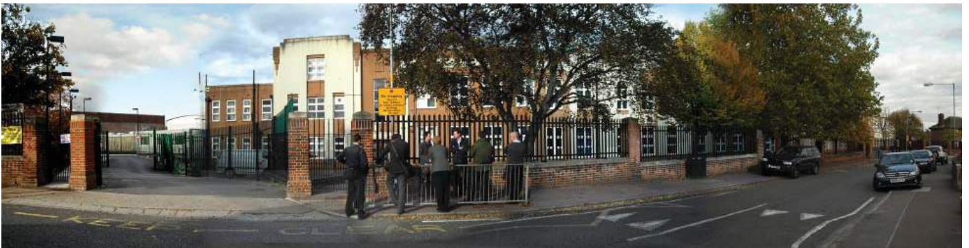
Existing frontage on School Road
