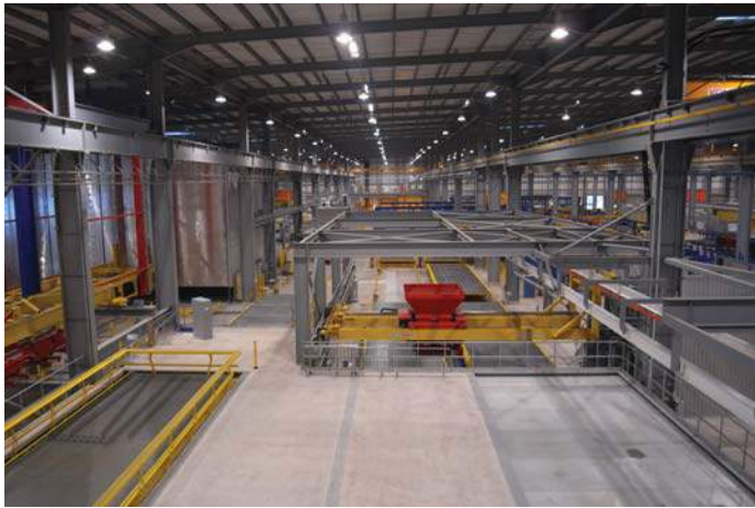
Laing O'Rourke precast concrete manufacturing facility
